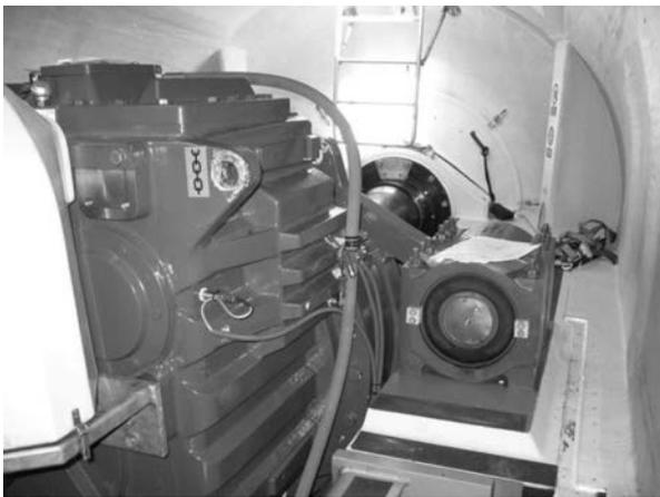
Fig. 3. View of the 1.5 MW wind turbine gearbox (front) and the main bearing (behind).
