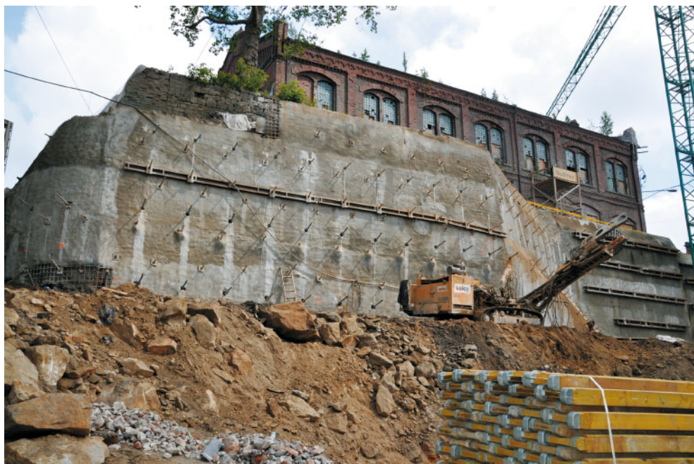
Fig. 9. Land mass and bath protection system – as of June 2012 (Photo by: A. Ostreġa)
