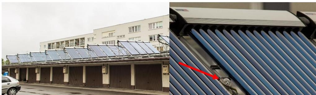
Fig. 1. Installation – left side, pyranometer mounted between pipes – right side
